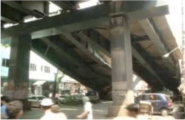
Figure 1: During casting period
