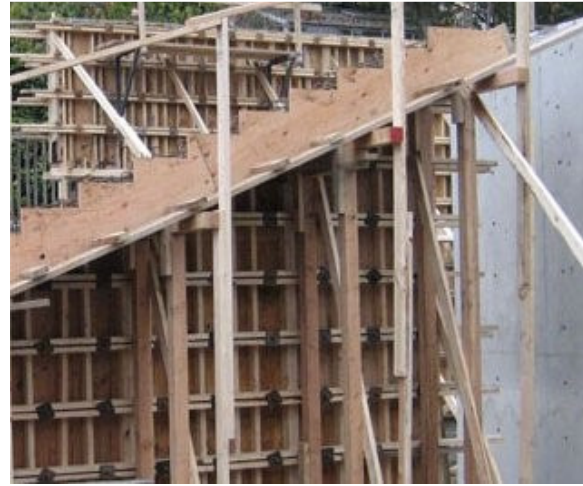
Timber formwork in staircase construction
