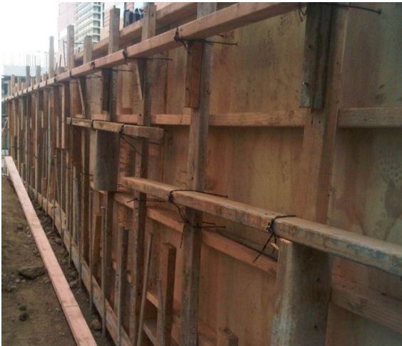
Plywood forms in combination with timber
