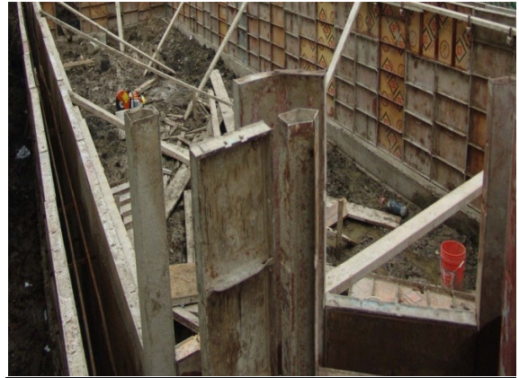
Steel formwork for RC Wall
