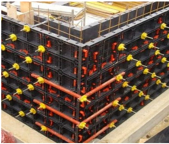
Plastic Formwork Concrete Wall
