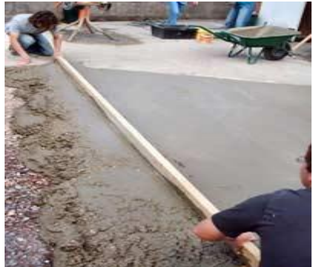
FINISHING OF CONCRETE SURFACE
