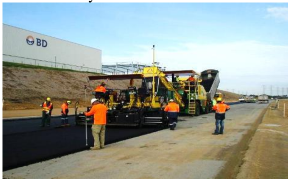
ASPHALT PAVER MACHINE
