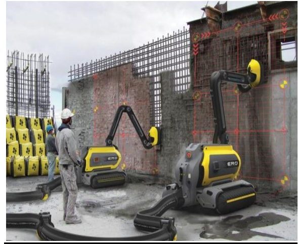
Use of ROBOTICS in infrastructure project
